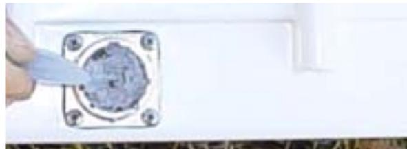
Figure 1 – Applying Silicon Dielectric Compound
